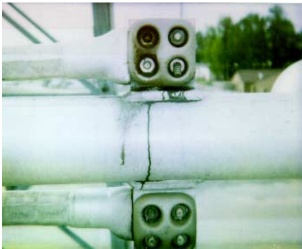
Figure 5 Photograph (left) and thermogram (right) of a severely overheated metal-to-metal connection
